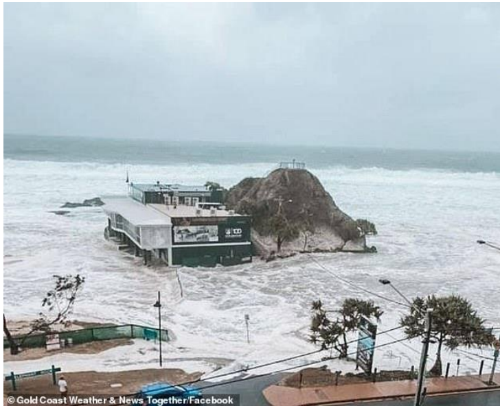
Currumbin SLSC rapid deterioration
